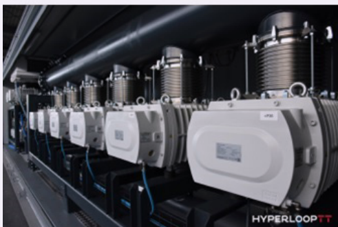
Fig. 4 a) HyperloopTT Vacuum System, b) Vacuum Pumps
